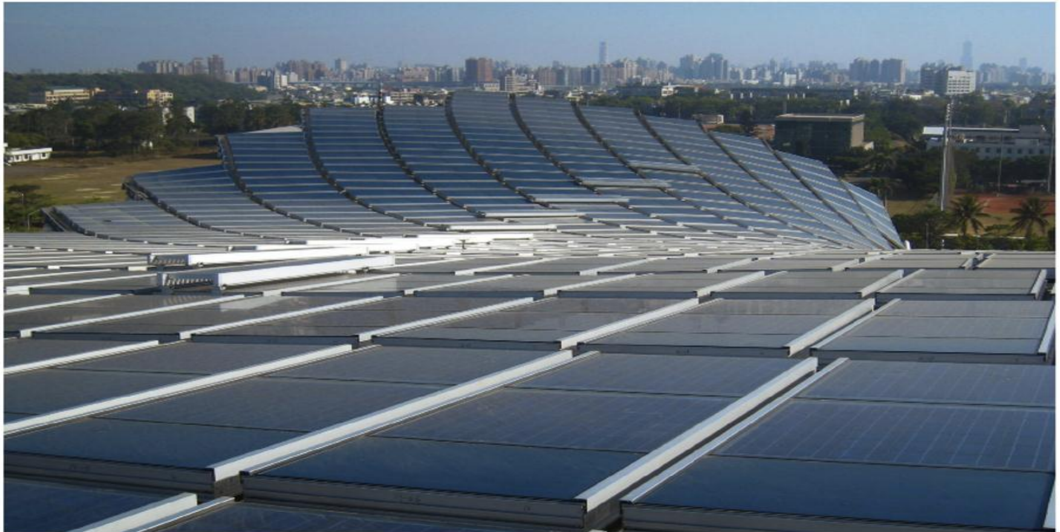
Each solar roofing component consists of two glass-glass modules, fitted with six by six polycrystalline cells. Different sizes can be achieved with the aid of an opaque edging strip.
