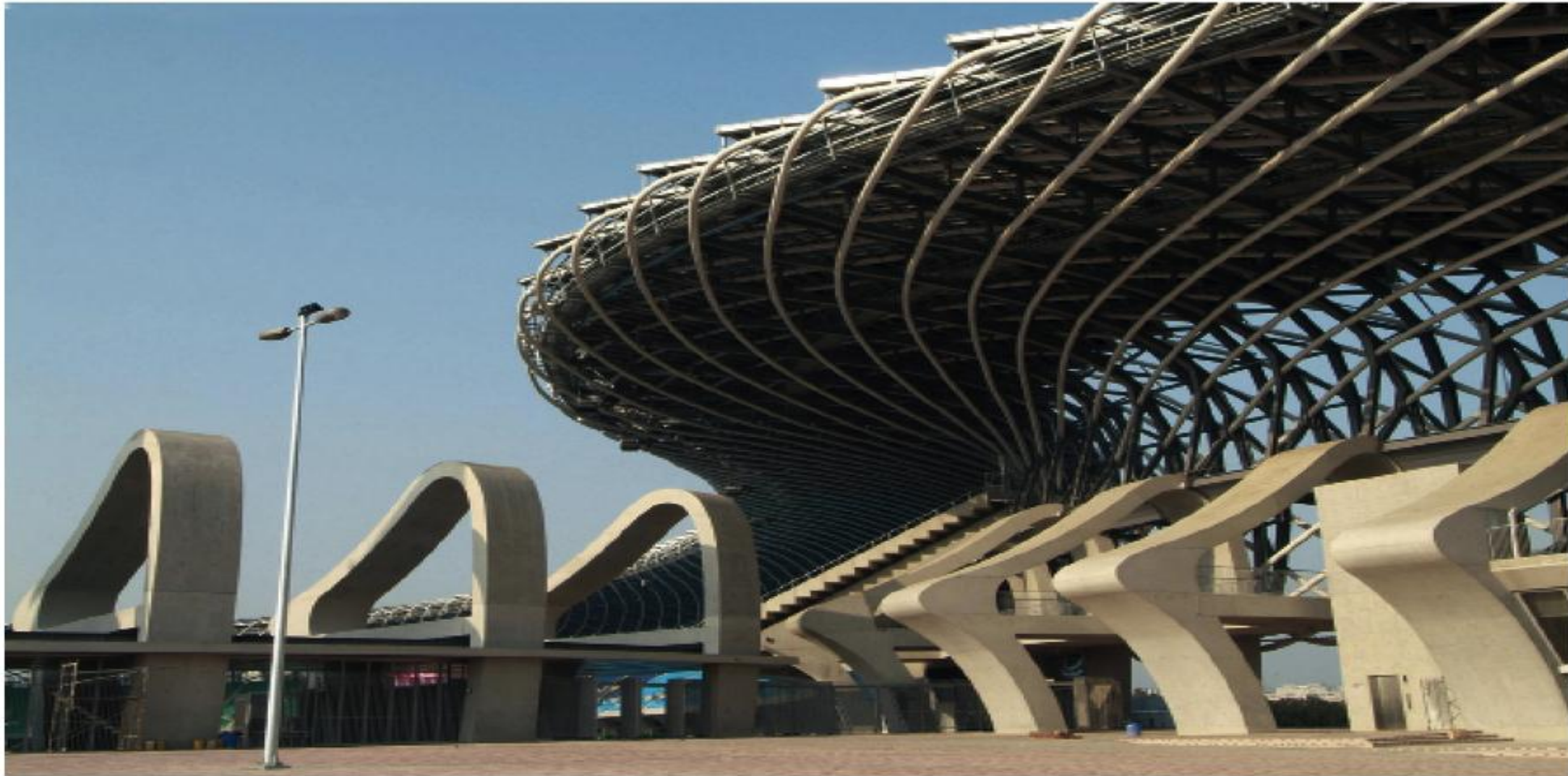
The framework struts carry the main load for the undulating roof. The spiral steel tubes take up temporary loads from earthquakes and wind.
